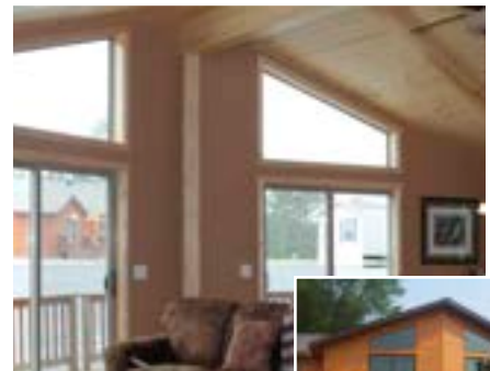
4/12 PARALLEL CHORD WITH KNOTTY PINE CEILING & PINE BOX BEAMS (Interior)
