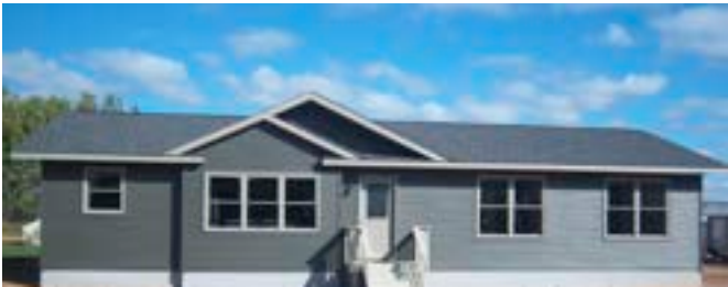
BOX BAY TO FLOOR OUTSIDE
