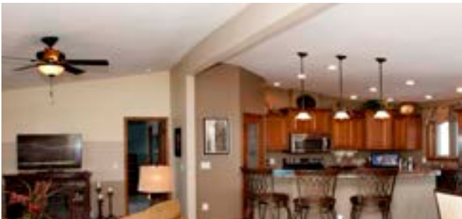
DRYWALL ARCHWAY WITH CATHEDRAL CEILING
