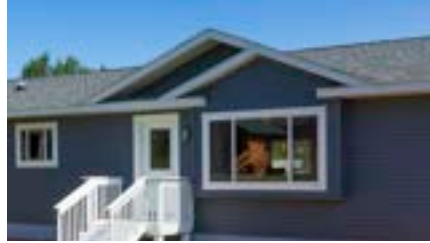
DORMER with Rake | Shingled Returns | Overhang Run-Through
